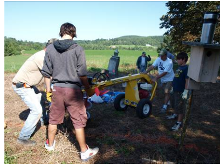
Auguring holes for the new fence
